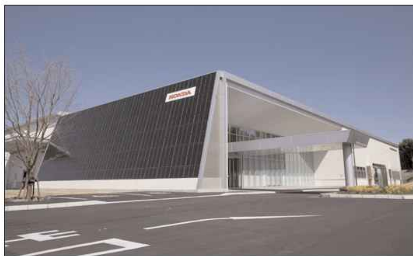
Figure 6. Honda's CIGS production facility.
